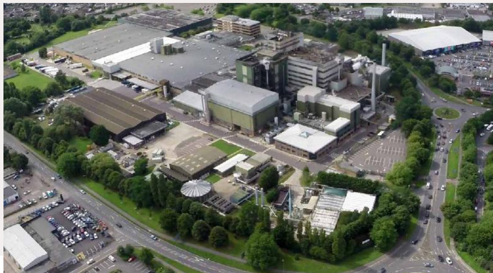
JDE manufacturing facility in Banbury, UK
